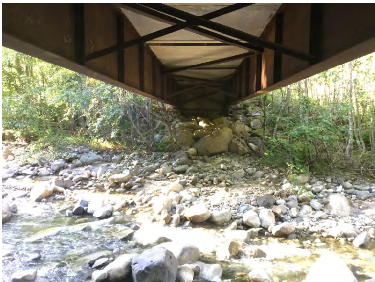
Left Bank Abutment when facing downstream
