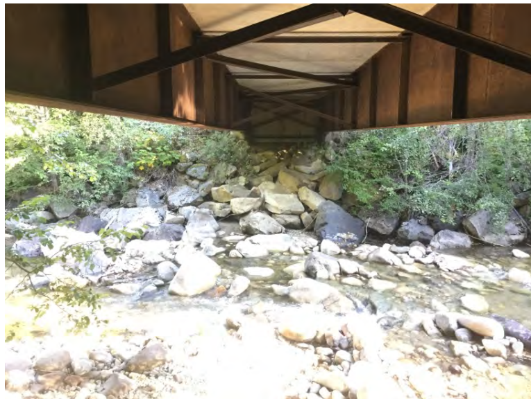
Right Bank Abutment when facing downstream
